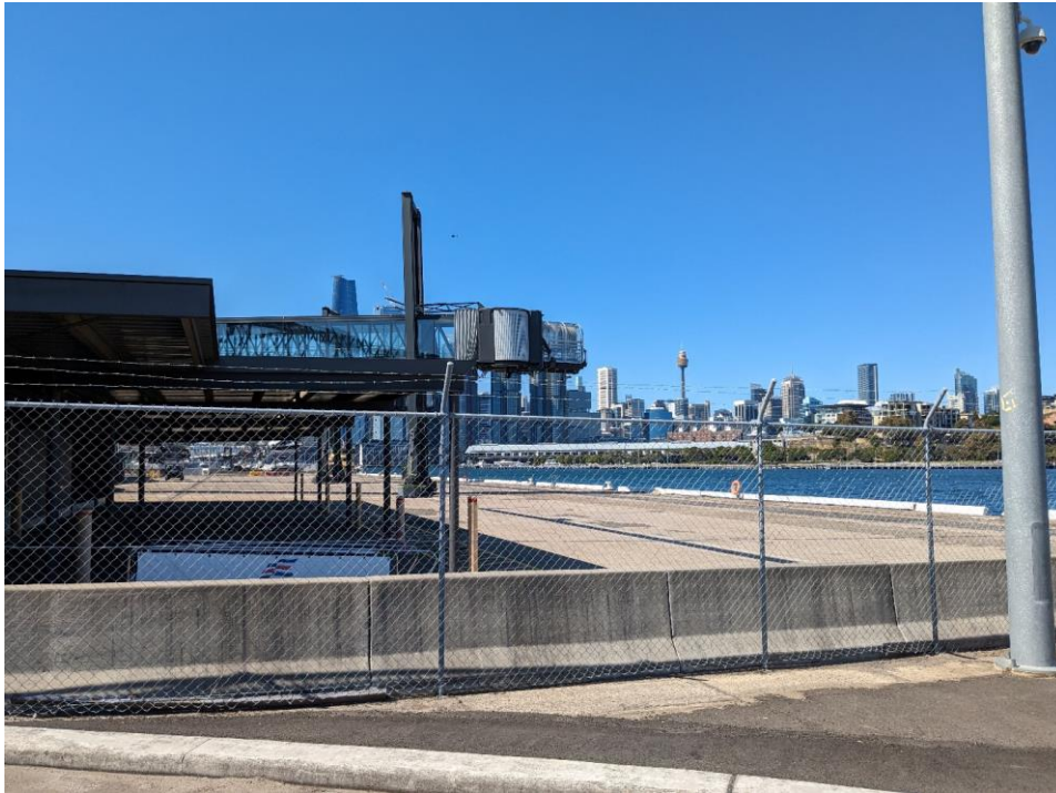
Figure 3-1 View looking east to White Bay 5 (Source: Worley Consulting, 2023)
