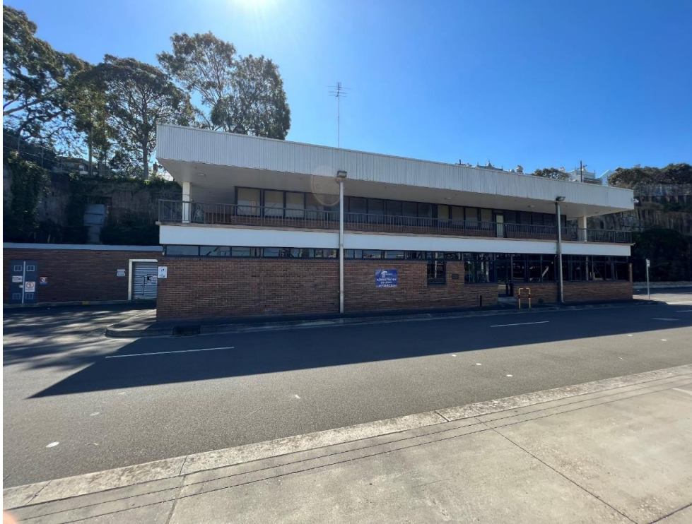
Figure 3-3 View looking north to the decommissioned White Bay 5 Administration Building (Source: Worley Consulting, 2023)
