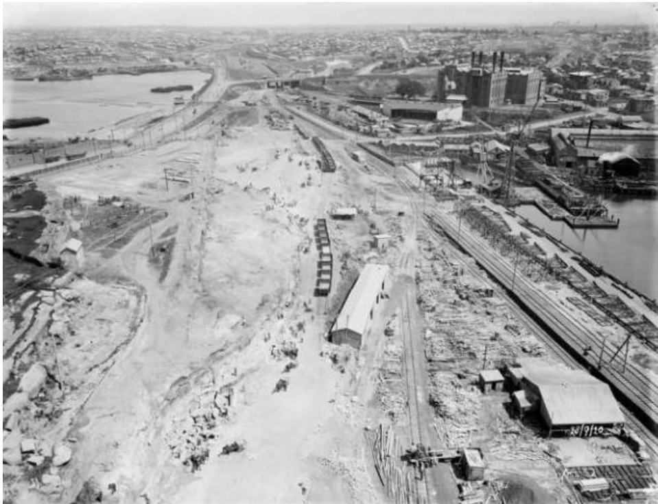
Figure 1-3 Quarrying at Glebe Island for Wheat Silos, undated (Source: State Library of New South Wales)
