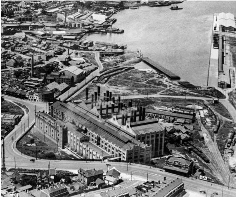
Figure 1-4 Aerial view of the White Bay Power Station circa 1930 (Source: City of Sydney archives, Graeme Andrews collection)
