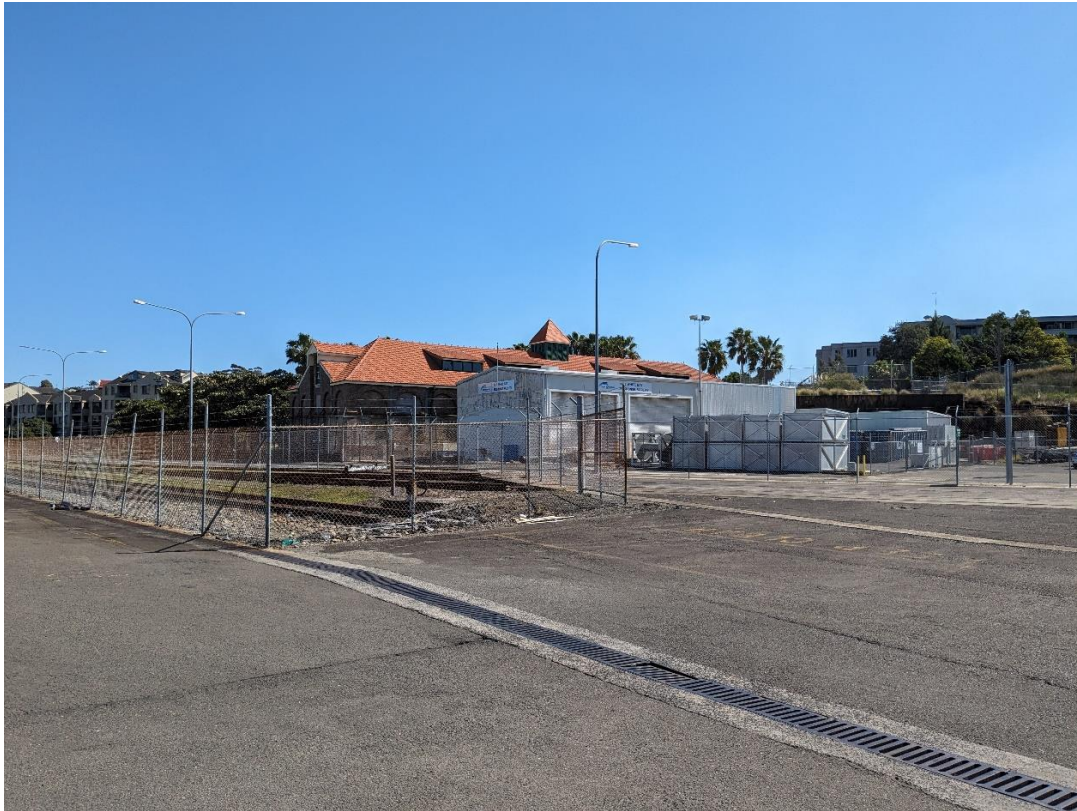
Figure 5-4 View looking west to administration buildings and remnant railway lines near White Bay 3 (Source: Worley Consulting, 2023)
