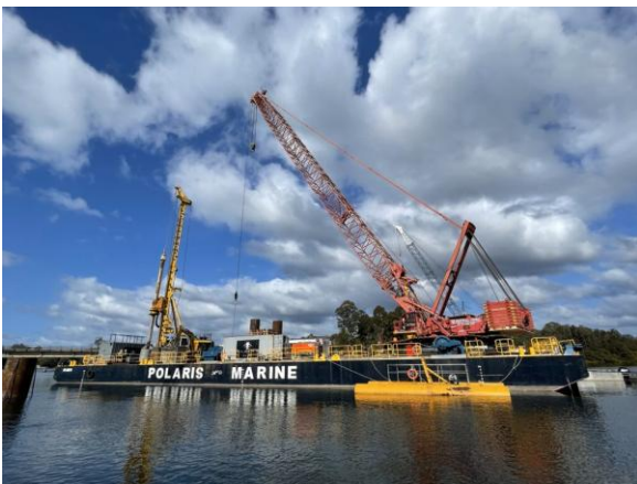
Figure 10: 53m PM East Crane Barge
