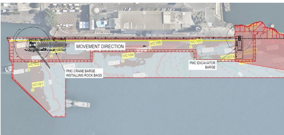
Figure 4: Crane barge placing scour protection from south to north
