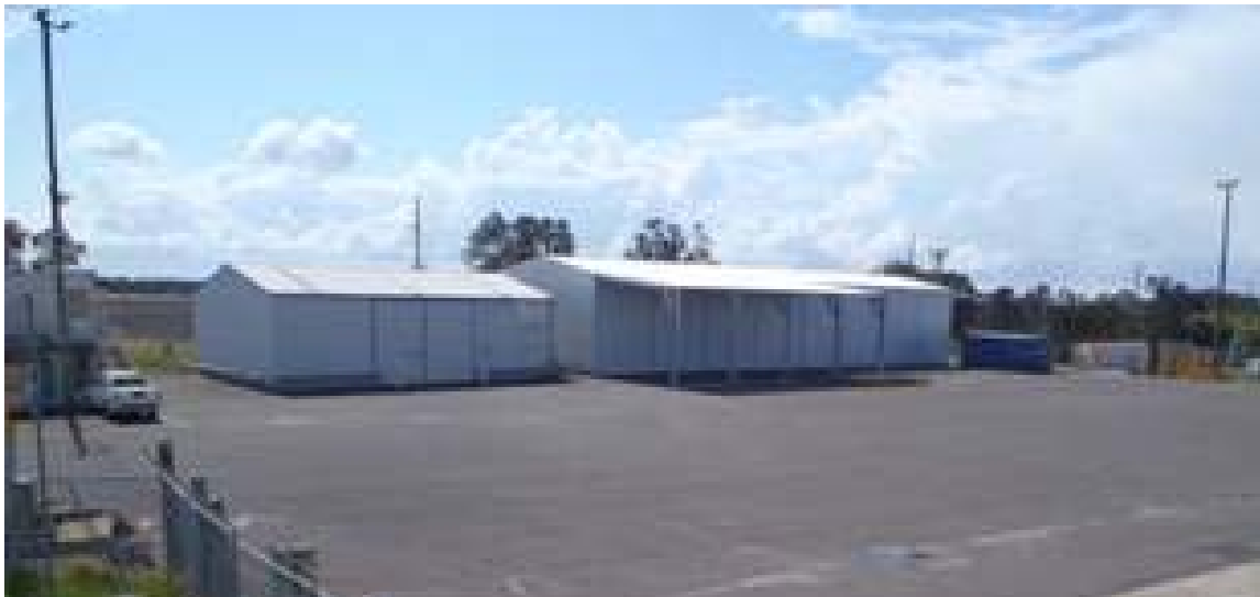
Goodwood Wharf – hard stand and lockable storage
