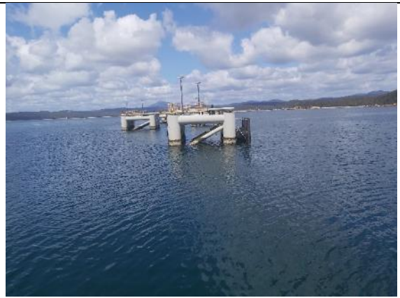
View of mooring and berthing dolphins
