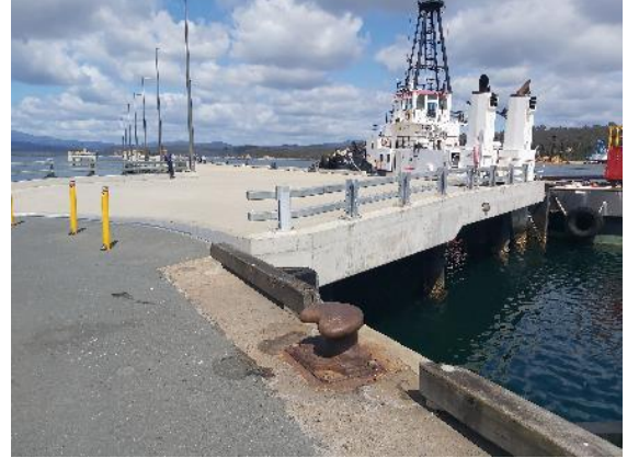
Showing point at which new wharf extension meets the existing breakwater wharf.
