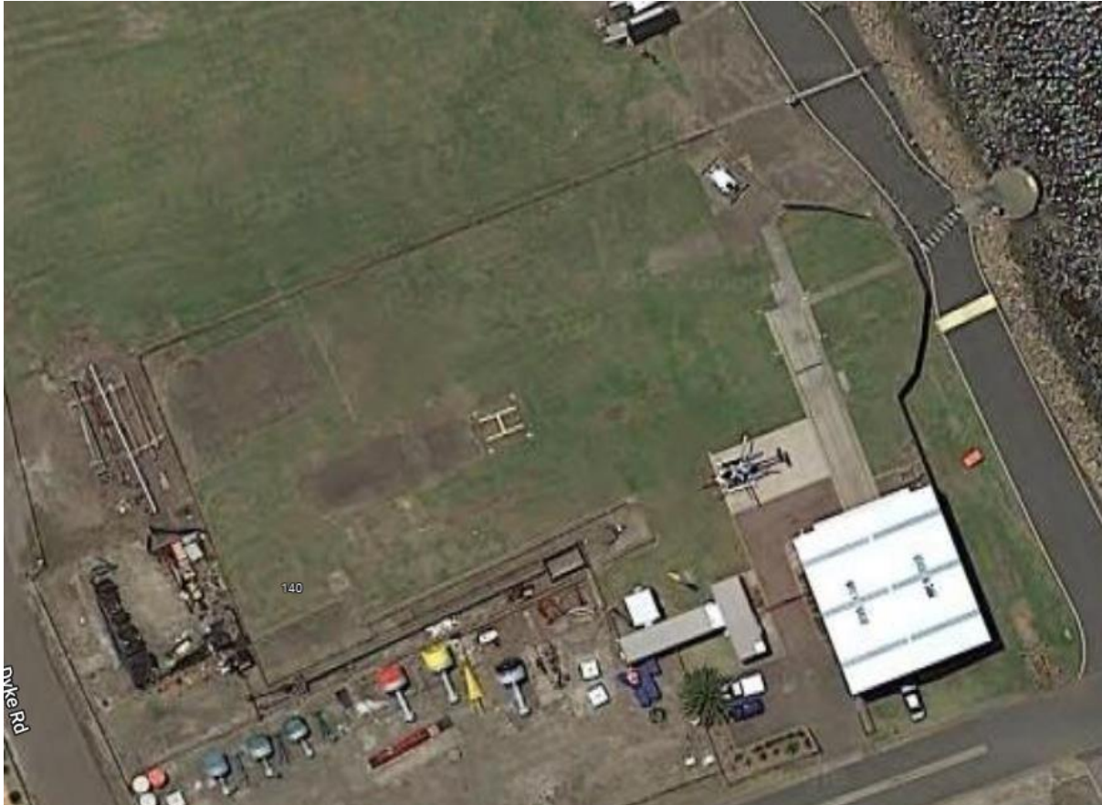
Fig 8 Dyke point Helipad overview
