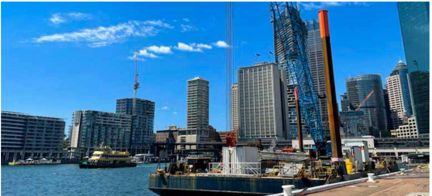
Berthing Infrastructure Project works, Circular Quay
