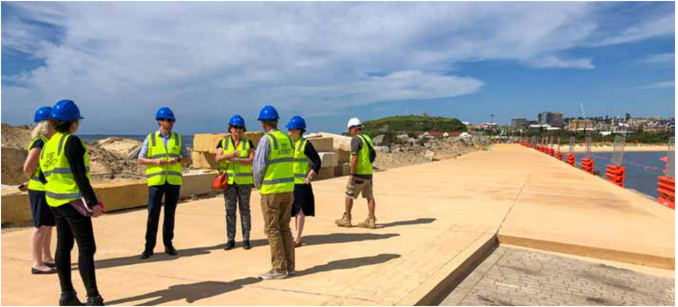
Inspecting progress of the Macquarie Pier revitalisation works, Newcastle
