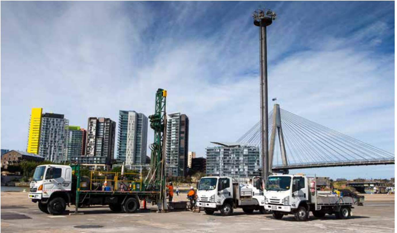
Bore drilling at Glebe Island for the Multi-User Facility
