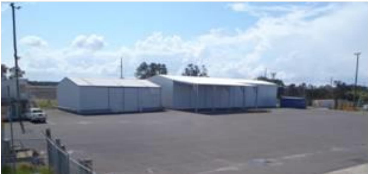
Goodwood Wharf – hard stand and lockable storage
