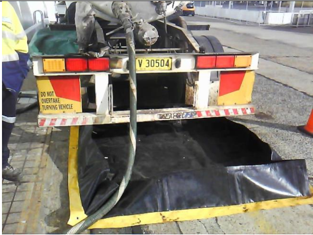
Photo 1 Transfer of oily waste (J120) from ship to tanker. Highly rated hose and connections and portable bund place beneath connection. Transfer was supervised.
