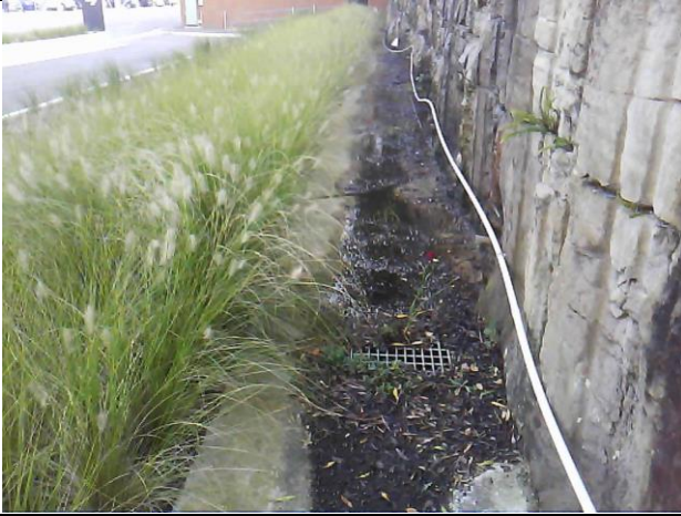
Photo 13 Landscaping near rock wall
