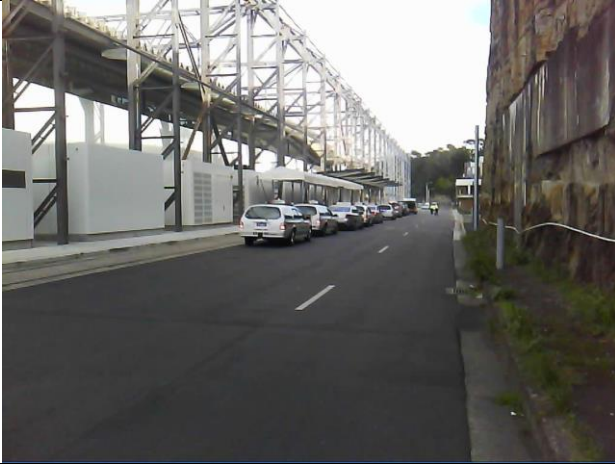
Photo 17 Railway tracks retained in taxi queuing area
