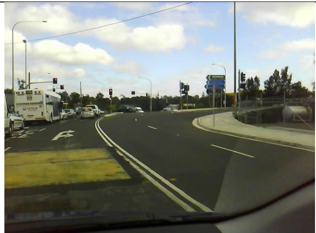
Photo 10 Intersection of James Craig Road and The Crescent showing right turn lane and signage
