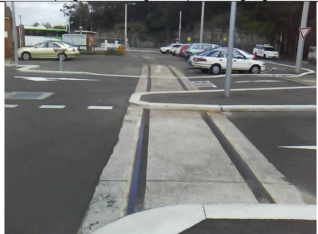
Photo 16 Railway tracks retained and incorporated into new carpark and road works
