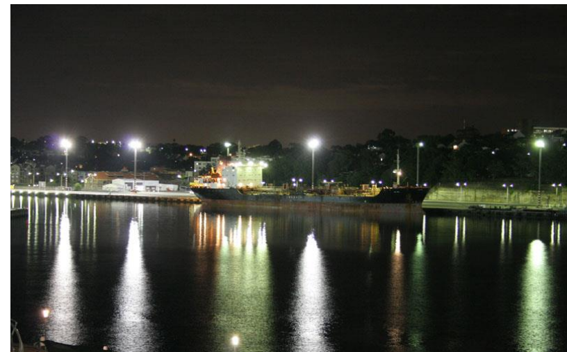
View from 2 Point Street towards the bulk liquids ship berthed at WB-4
