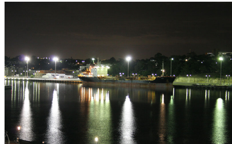
View from 2 Point Street towards the bulk liquids ship berthed at WB-4
