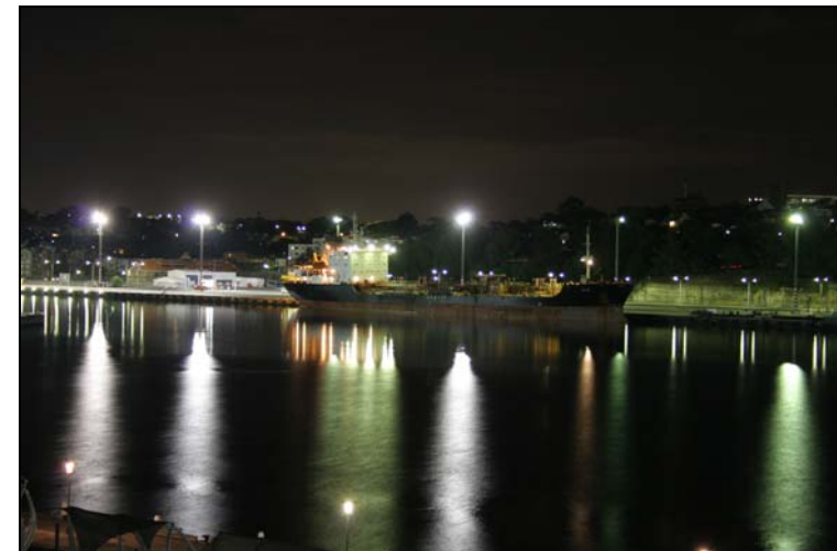
View from 2 Point Street towards the bulk liquids ship berthed at WB-4
