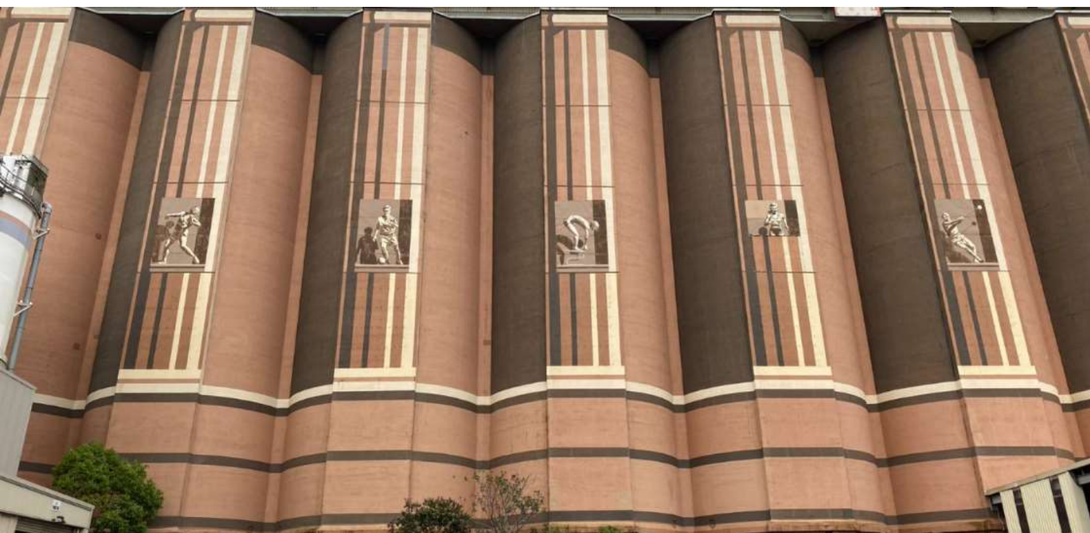
Figure 5: Glebe Island Silos, Zach Nix – NBRIS, 2022
