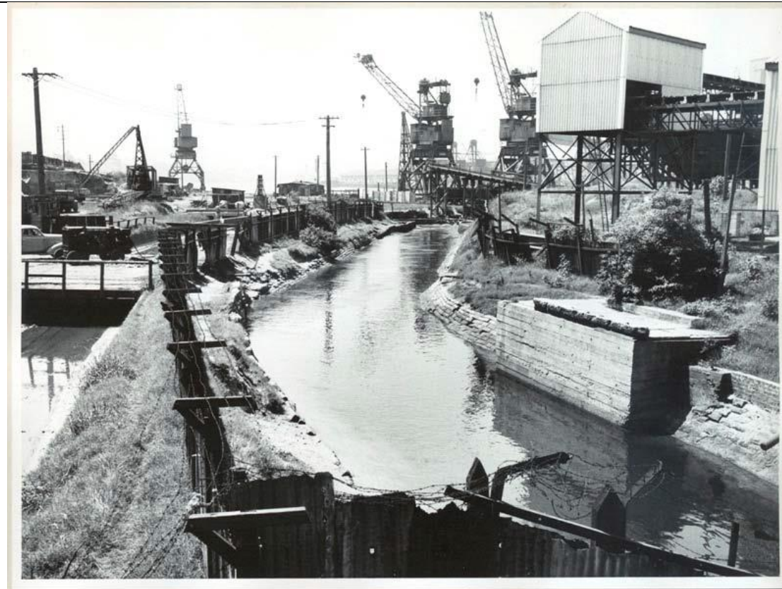
Caption: View of the what appears to be the original cooling water canal looking northeast
