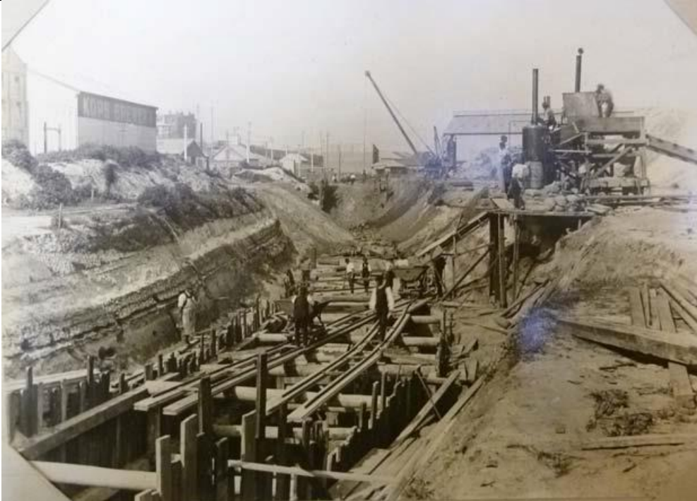
Caption: View of what appears to be the conversion of the west section of the cooling water canal to a conduit
