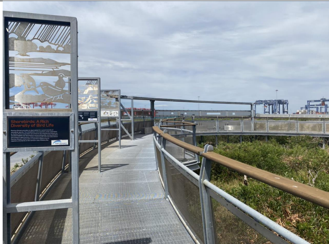
Caption: Viewing platform providing public visual access to Port Botany Old Government Wharf Remains and Penrhyn Estuary
