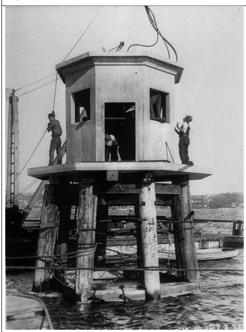
Caption: Georges Head [sic, Western Channel Light], precast top being placed on pile foundation
