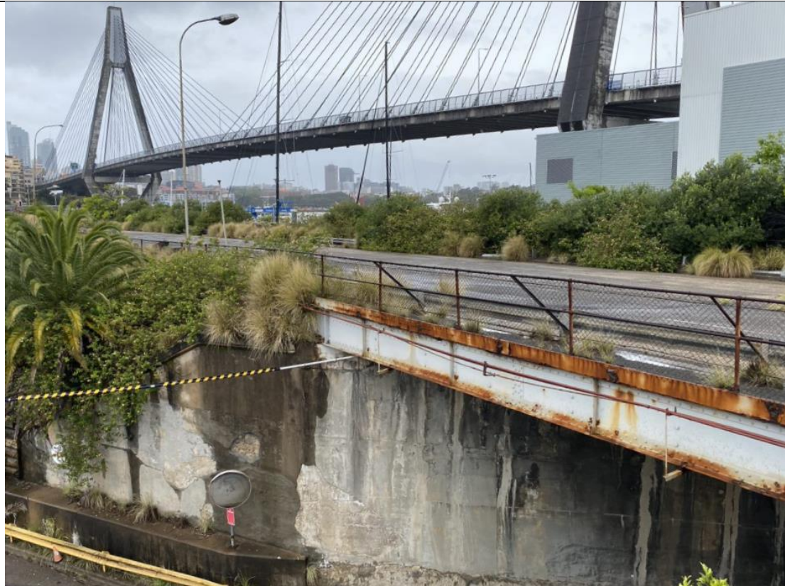
Caption: Glebe Island Bridge approach closeup from Monument Lookout
