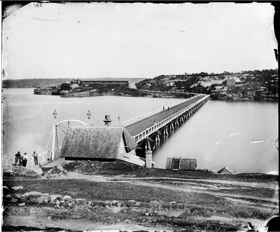
Caption: Blackbutt Bridge [first Glebe Island Bridge]
