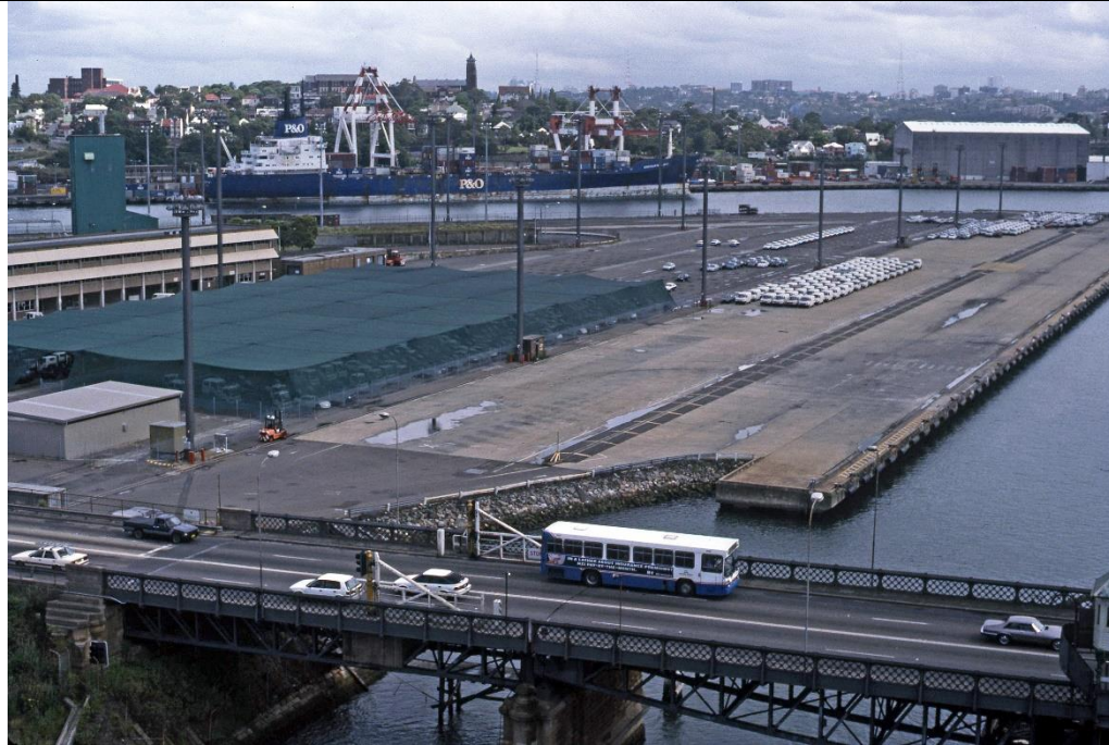
Caption: View of the Glebe Island Bridge the day before the opening of the new Anzac Bridge with the P & O cargo ship Encounter Bay moored at White Bay
