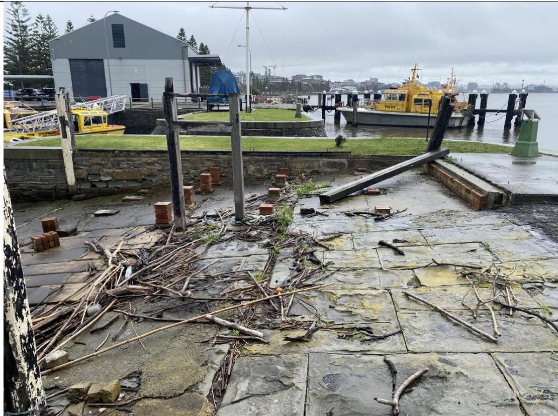
Caption: Location of former boat shed / slipway, piers visible
