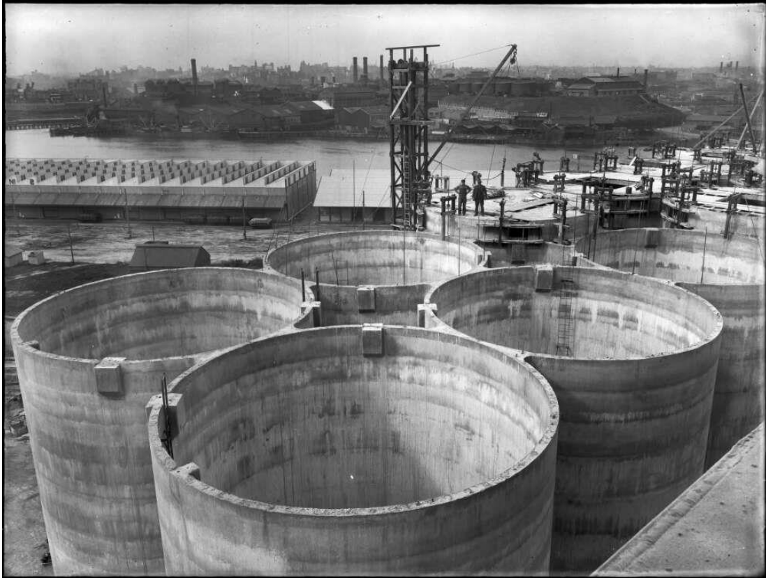
Caption: Silo construction, Glebe Island
