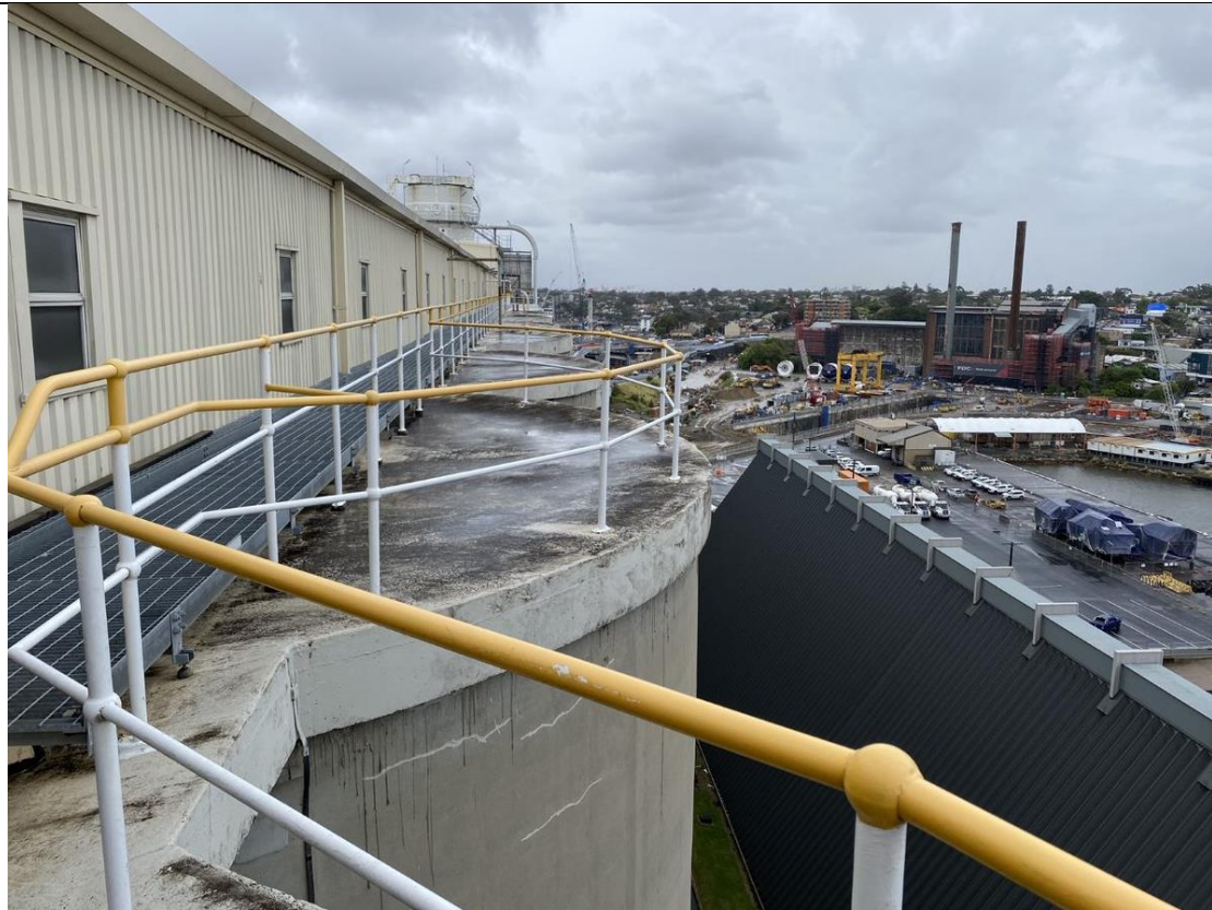
Caption: Top of Glebe Island Silos, looking northwest
